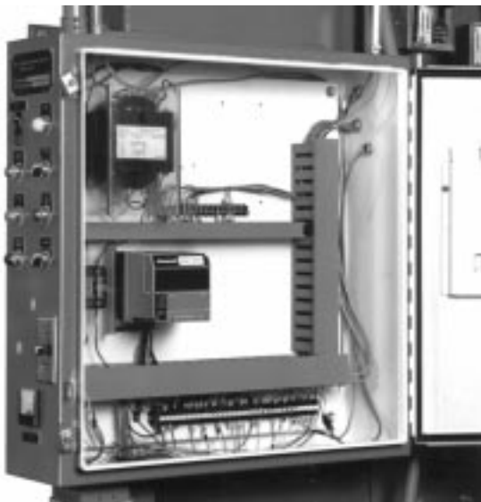
Fig. 9—Electrical panel installation.
